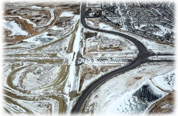
17 Avenue SE and Stoney Trail SE
