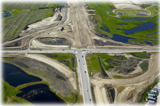
17 Avenue SE and future Stoney Trail SE July 2011
