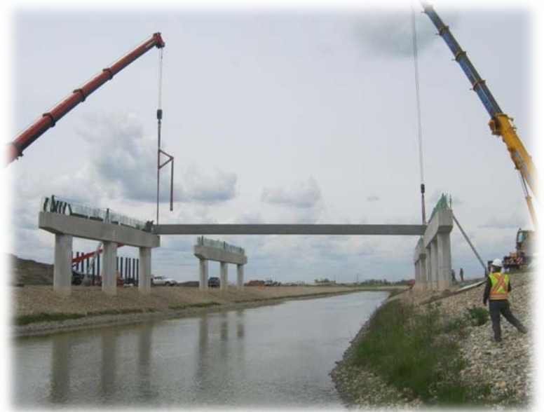
First bridge girder installation at the WH Canal May 2011.
